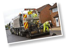
This type of cold treatment is called microsurfacing, it only takes about half an hour to set hard. The new surface consists of two layers, it helps to waterproof the road to prevent ice from causing cracks and potholes. You can use the road again soon afterwards. If it rains before or during the work, we may have to delay it, or come back to do the second layer later. The dates displayed on the signs will be changed so please check these regularly.
