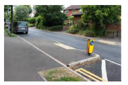
The build-out design must include a physically protected cycle bypass lane of at least 1.5m width unless it has been designed in association with pedestrian crossing facilities. Or if this is not achieveable, an unprotected cycle lane of over 1.5m. Or if this is not achieveable a maximum running lane width of 3.0m.
