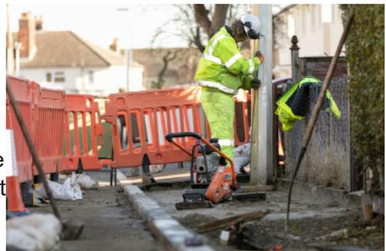
New footways are designed to be at least 1.5m wide to accommodate wheelchairs and parents with children etc. In circumstances where there is minimal usage this can be reduced to an absolute minimum width of 1.2m.
