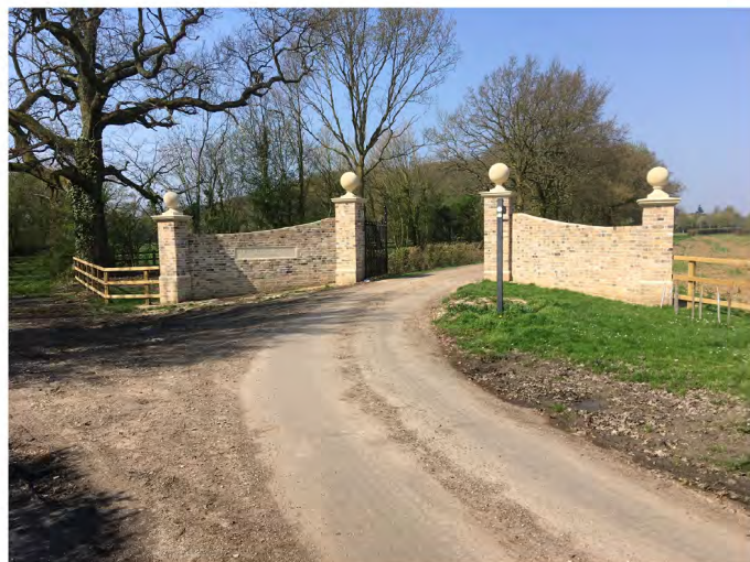
East Gate - Gate opening & brick piers
