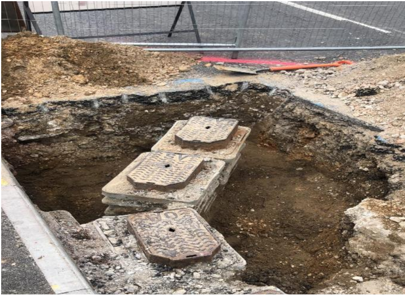
Ipswich Road South Anglian Water valves dug out for final testing in this area.
