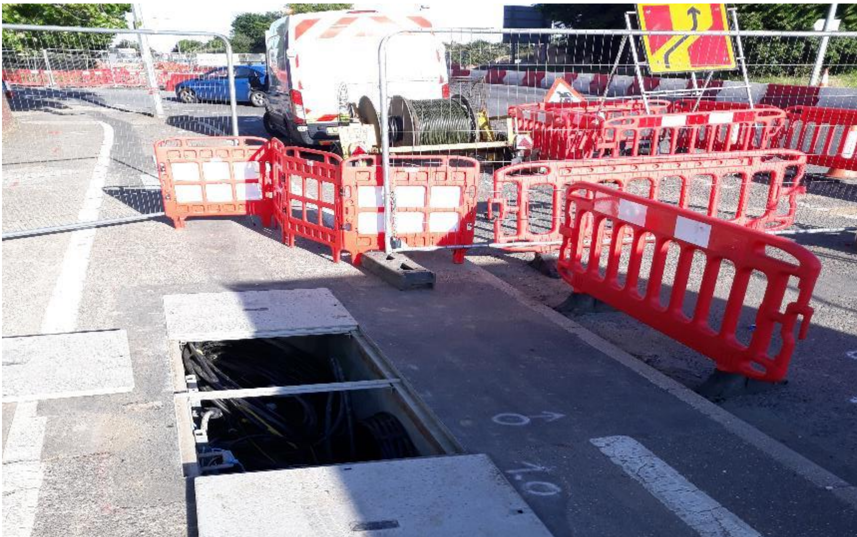
Cabling for BT Openreach in Construction Zone 1C. This is ongoing works for fibre and copper diversions.
