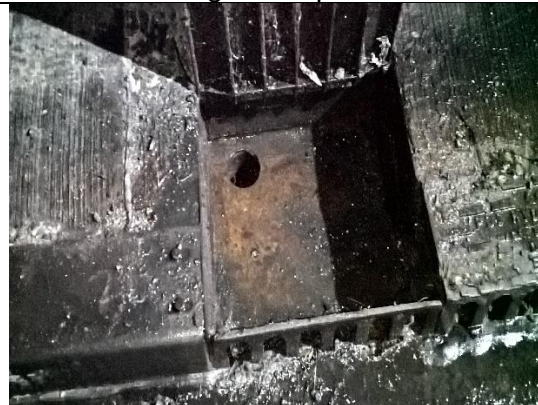
After drainage clearance photo
