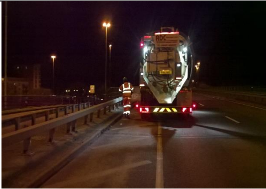
During works photo 1
