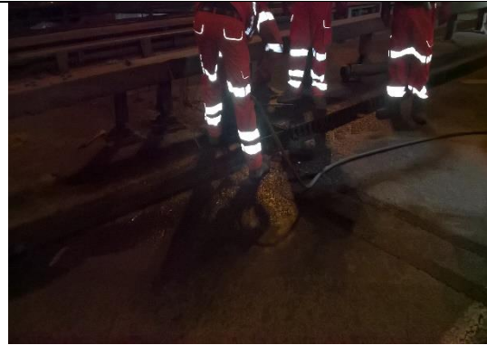
During works photo 2
