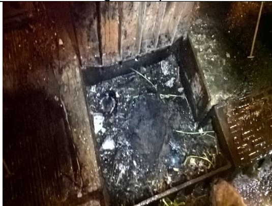
Before drainage clearance photo
