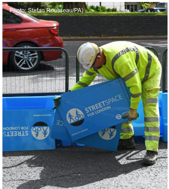
A worker puts the finishing touches to a pop-up cycle lane on Park Lane, London
