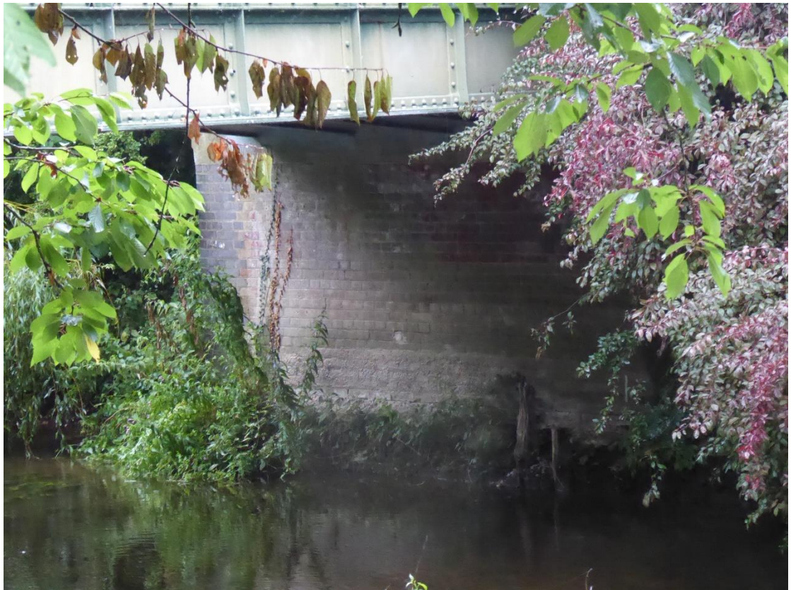
Figure 12: View of bridge abutment
