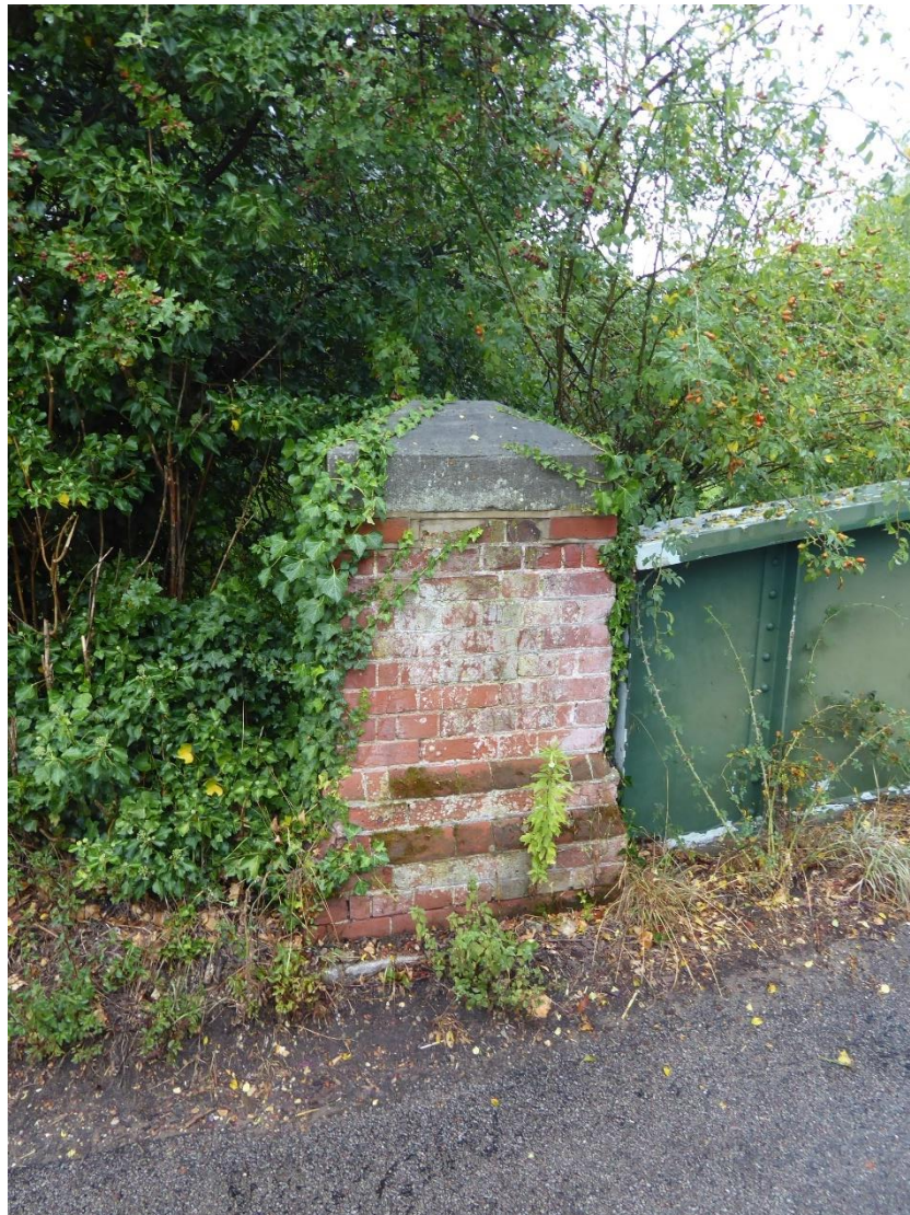
Figure 10: View of brick and granite pier
