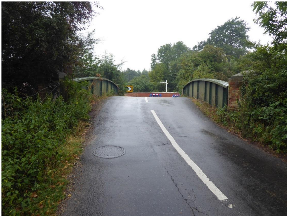
Figure 9: View of bridge from north side
