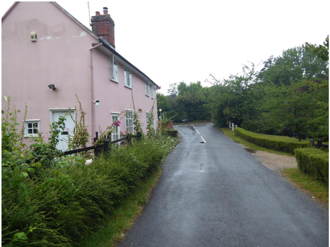
Figure 13: View of Island Cottage
