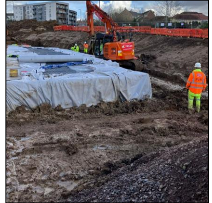
Installation of attenuation tank
