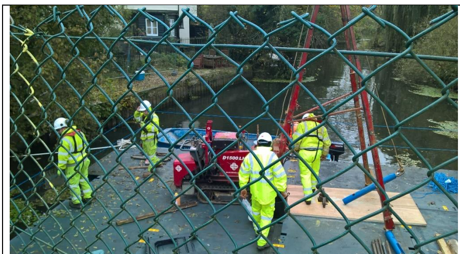
Borehole testing work
