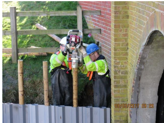
Bamboo Being installed Photo
