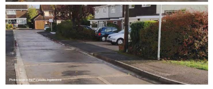
Essex has many miles of concrete roads, particularly on estates built decades ago. Concrete roads can last for many years, but eventually the slabs start to move and/ or crack and break. Replacing sections, or doing large concrete patches, is very expensive.
