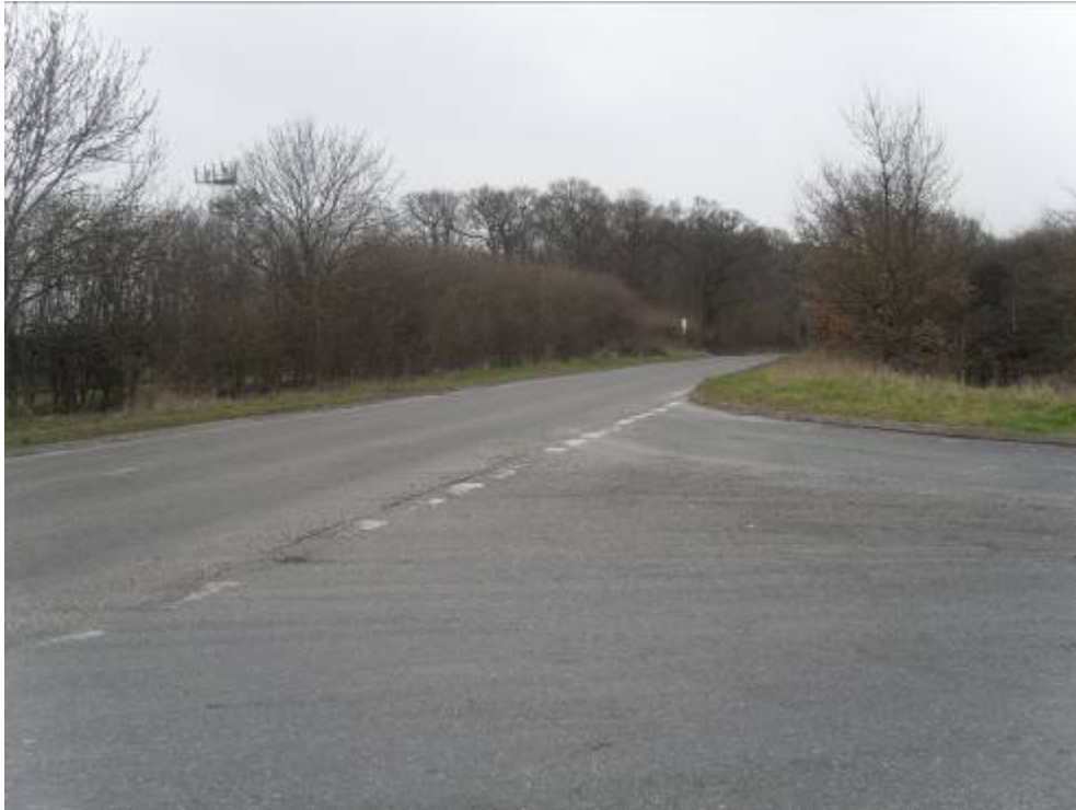
Photo 2 – Give way road markings badly worn.
