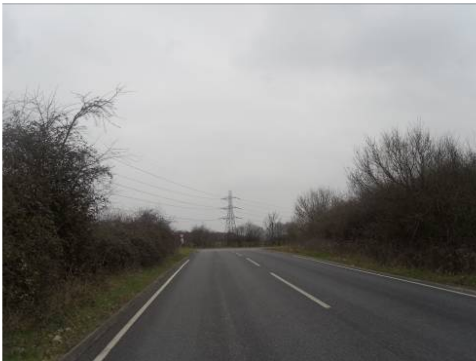
Photo 1 – Junction is inconspicuous on the Wrightsbridge Road north-west bound approach.
