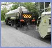
**Micro surfacing** is a slightly more durable and more expensive process which places a thin layer of a completely new surface on the road.
