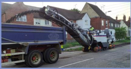
**"Insitu-recycling** is only used in limited areas where the road is very badly out of shape. A very durable new surface can be laid, and logistics make it easier to re-use existing materials rather than bring in new stone. It is marginally more expensive treatment per area covered than resurfacing or other treatments."
