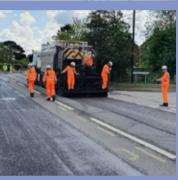
**Machine resurfacing** is where the existing surface is removed, and completely new depth of surface is laid as a replacement. It is a more expensive and slow process but is a great treatment to use in places where the road is badly worn and is required to take heavy traffic.
